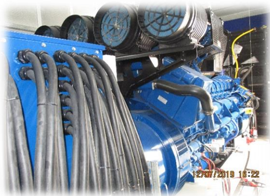
The Standby Emergency Generators & engines inside the acoustic enclosures at The Royal Glamorgan Hospital
