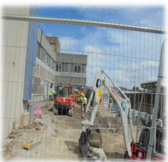
PCH Phase 1B external ground works
