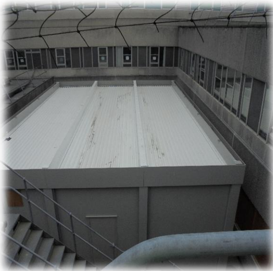
PCH Phase 1B new offices, storage & staff changing area
