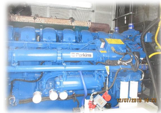
The Standby Emergency Generators & engines inside the acoustic enclosures at The Royal Glamorgan Hospital
