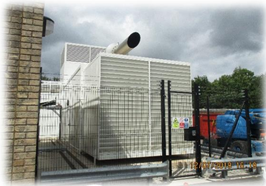
2 Standby Emergency Generator acoustic enclosures at The Royal Glamorgan Hospital to provide electrical site resilience
