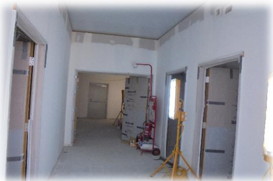
PCH Phase 1B works prior to the ceiling installation
