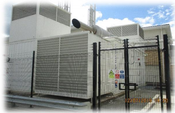
2 Standby Emergency Generator acoustic enclosures at The Royal Glamorgan Hospital to provide electrical site resilience
