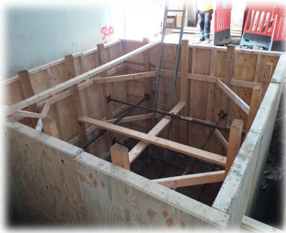
PCH Phase 1B works creation of a new lift pit into the ground i.e. below ground floor level
