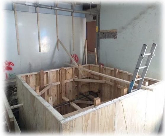
PCH Phase 1B works creation of a new lift pit into the ground i.e. below ground floor level
