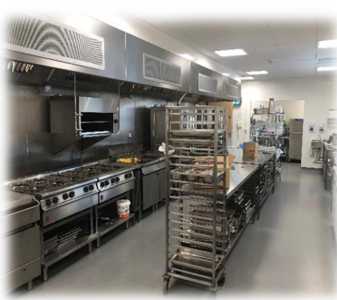
PCH Restaurant food preparation area
